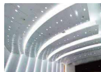
Ceiling curtain wall
